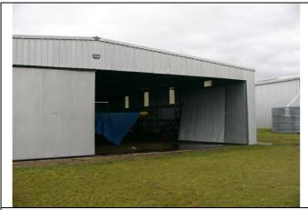
Above photos show damage to the QUA Hangar. Main damage is to the doors, fittings and some side wall panels. Photo on the right shows the remains of John and Tanys's unfortunate hangar with rolled up Drifter remnants below. The Drifter was destroyed. Bottom right photo shows the wing of a Tiger Moth clipped by a door on the vintage hangar. The doors at the other end were blown off. The QVAG Clubhouse suffered roof damage from the flying debris.
