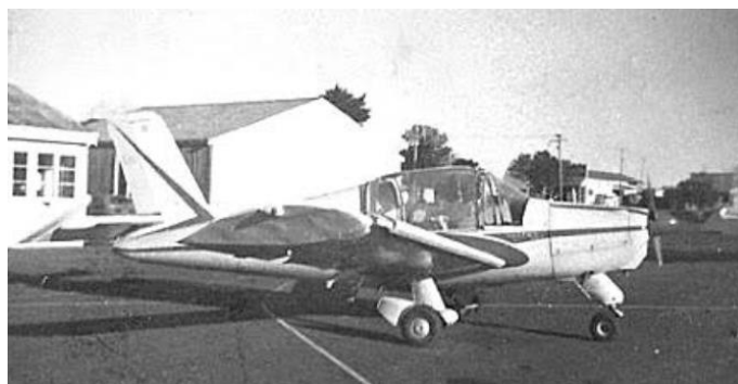
CBT on the apron at the Northland Districts Aero Club in 1963. The starboard automatic leading-edge slat can be clearly seen.
