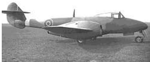
Gloster Meteor DD206/G was the first Meteor to fly, on 5 th March 1943. It used the Whittle W.2 engine.
