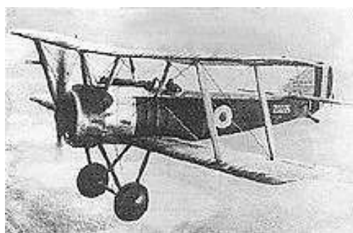
Tom Sopwith's "Pup" with its 80 hp L Rhone engine. Much loved by RNAC and RFC pilots alike.
