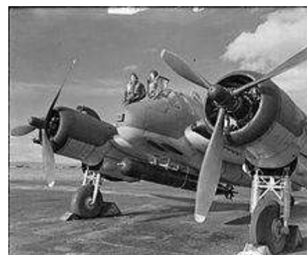
Mk V1C "Torbeau", with an 18inch torpedo
