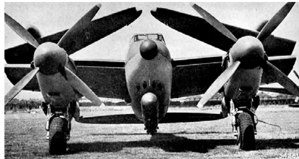
Folding wings and a torpedo fitted out the "Sea Mosquito"
