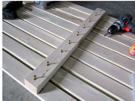
Centre braces screwed in place
