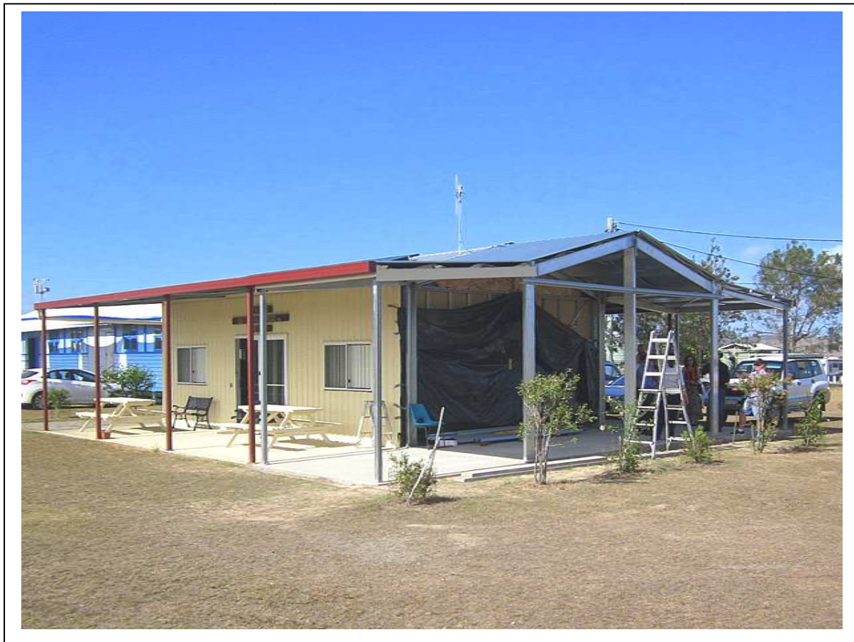
The extensions to the BVSAC Clubrooms underway (See pg 3).
